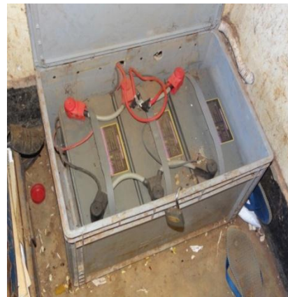
Battery box with rubbish at Katine SS in Battery and surrounding area coated with dust at Soroti District. Agwate SS in Dokolo District
