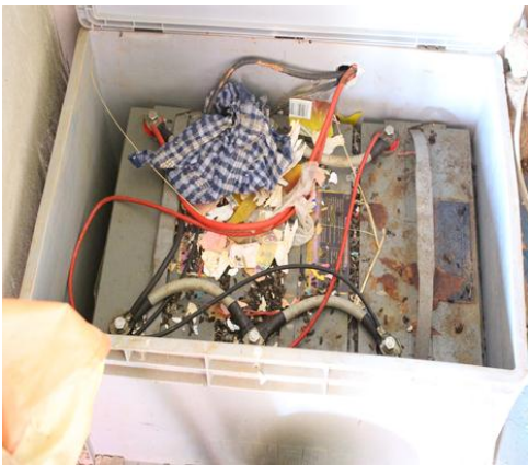
Battery box with rubbish at Katine SS in Battery and surrounding area coated with dust at Soroti District. Agwate SS in Dokolo District
