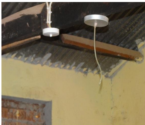
Vandalized Lamp Holders at Kangai S.S.S in Dokolo. Battery was stolen from the battery box at Nakalama S.S. In Iganga
